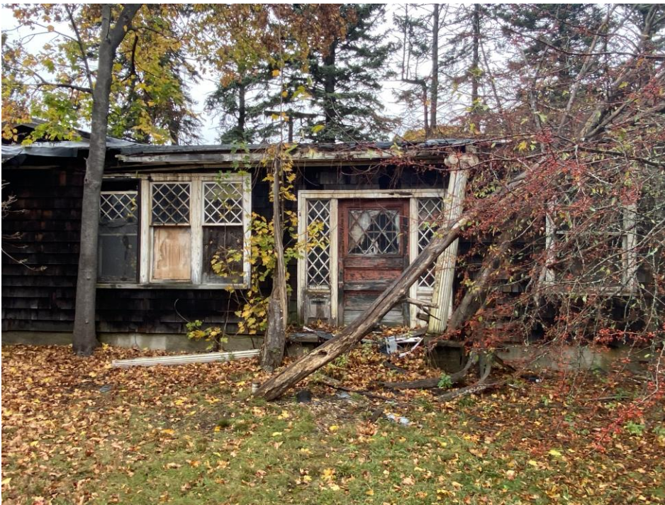
Little House rear ell, SE wing, from S.
