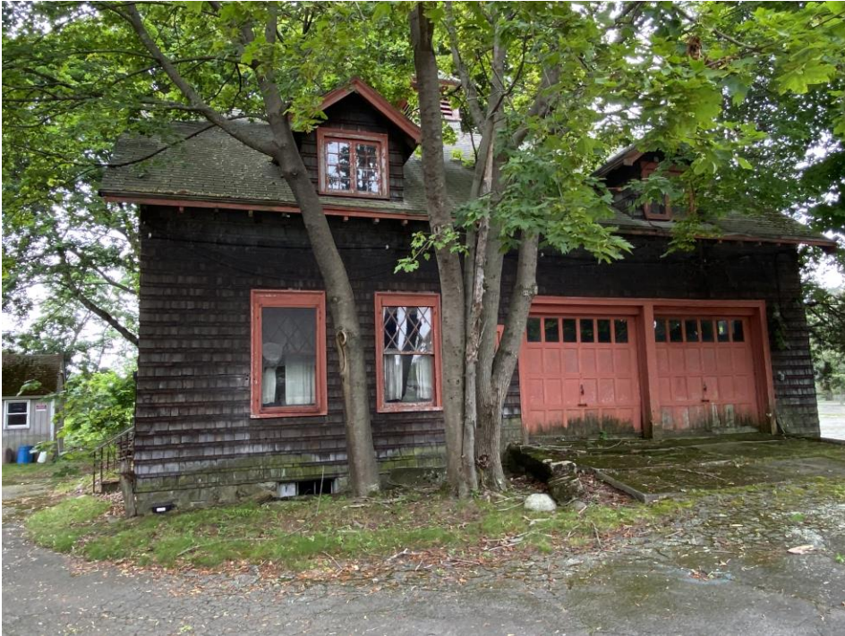
Little House barn1 from NW.
