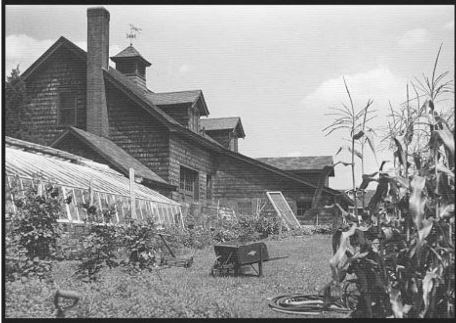
Little House barn 1 from S. (Swampscott Public Library)
