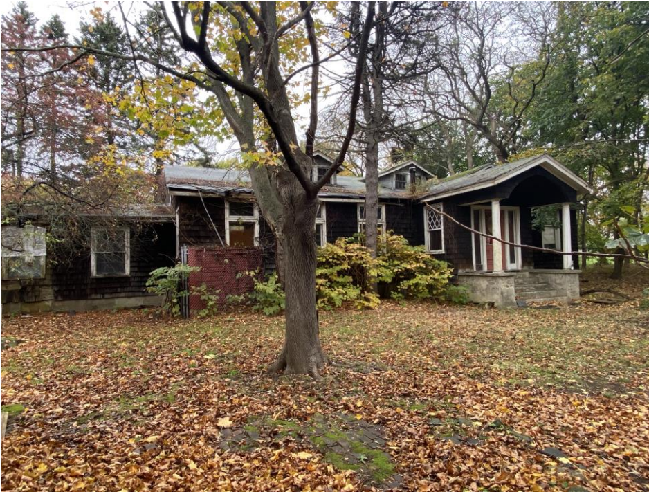
Little House bungalow from SW.
