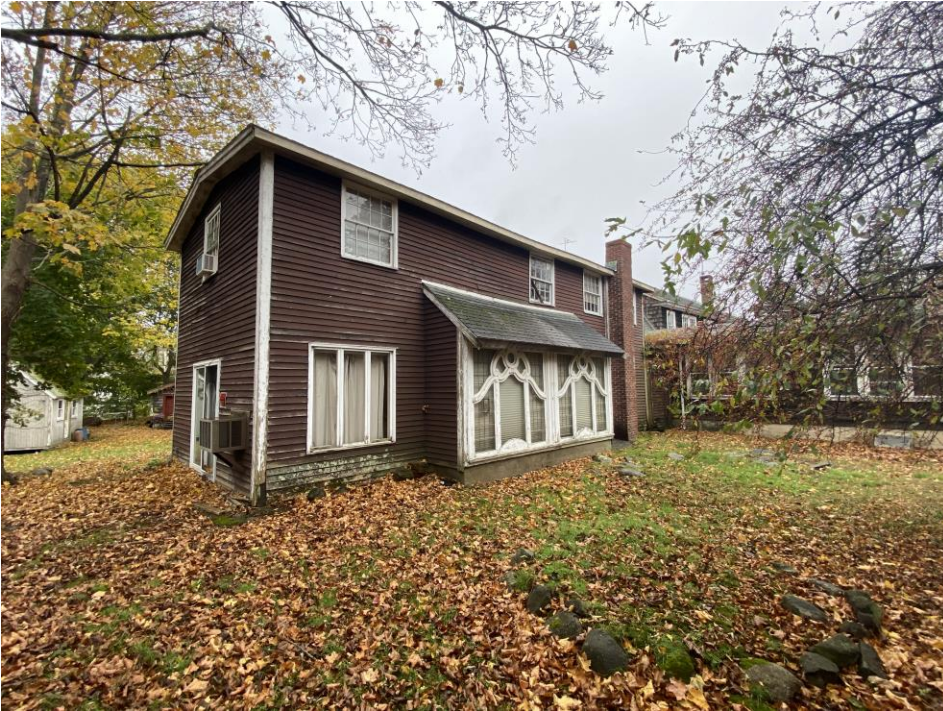
Little House barn 2 from NE.
