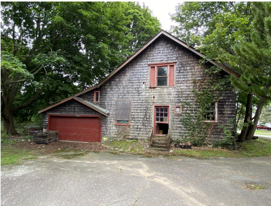
Little House barn 1 from NE.
