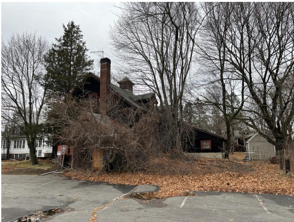
Current image of Little House barn 1 from S.
